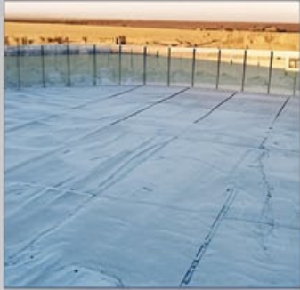
Erricson Dam IPV Cement Dam
