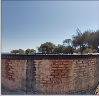
DIY Cement Dam
