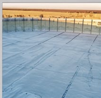
Erricson Dam IPV Cement Dam
