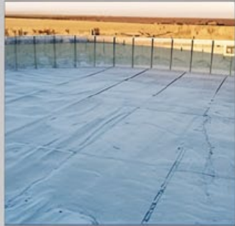
Erricson Dam IPV Cement Dam
