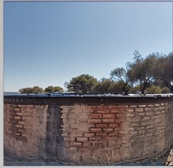
DIY Cement Dam
