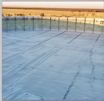
Erricson Dam IPV Cement Dam
