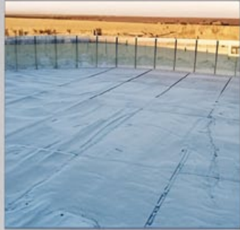
Erricson Dam IPV Cement Dam
