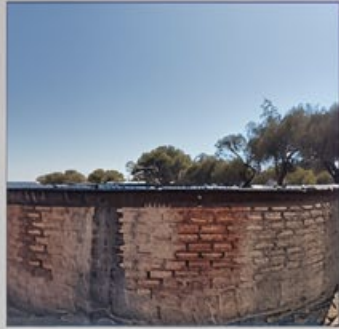
DIY Cement Dam
