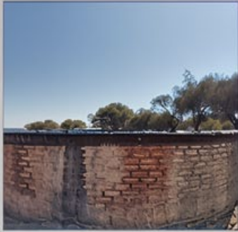
DIY Cement Dam
