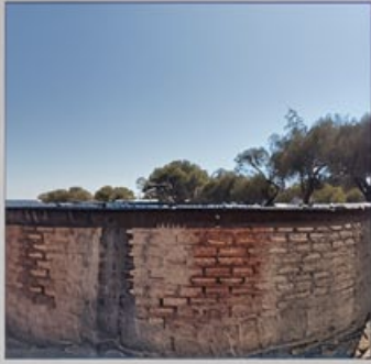
DIY Cement Dam
